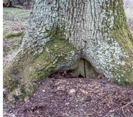
Opening at bottom of tree
